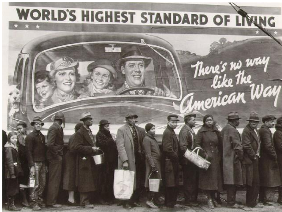
Flood Relief Line in Louisville, KY (Credit: Margaret Bourke-White, 1937)
